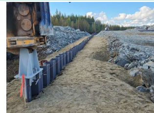
Installation des palplanches B2 S-O
